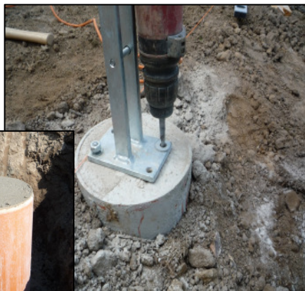
5. Pfostenfuss Bohren
